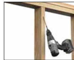
STUD TO DOUBLE TOP PLATE
