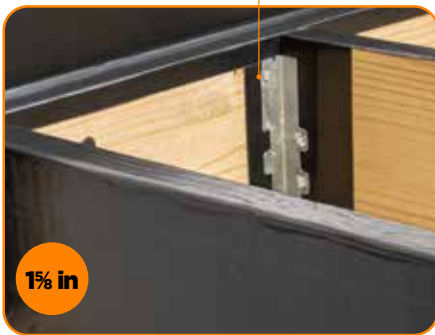
A BETWEEN JOIST HANGERS AND LEDGER BOARD
