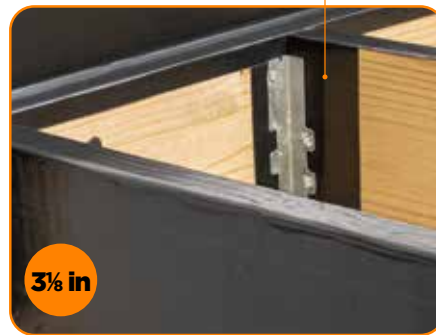
B BETWEEN FRAMING AND JOIST HANGERS
