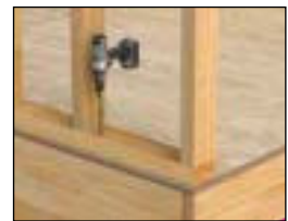
SOLE PLATE TO RIM BOARD CONNECTIONS
