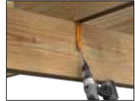
DECK JOIST TO BEAM
